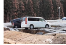
Quake soil liquefaction damage in the parking lot at the Shirakawa Plant
