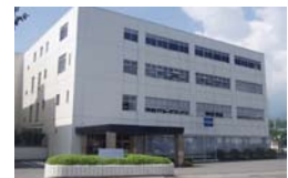
Repair Center (Nagano, Japan)
