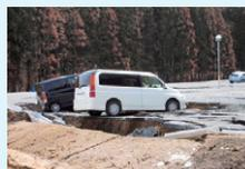
Quake soil liquefaction damage in the parking lot at the Shirakawa Plant
